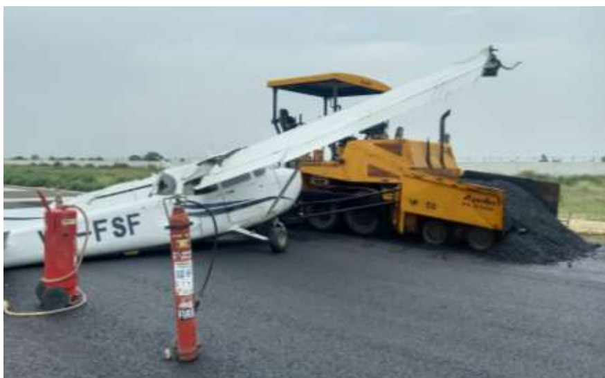
Figure 13: Freshly laid surface and paver machine loaded with asphalt
