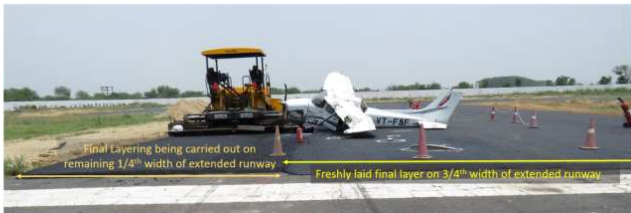
Figure 8: Status of work on the extended runway
